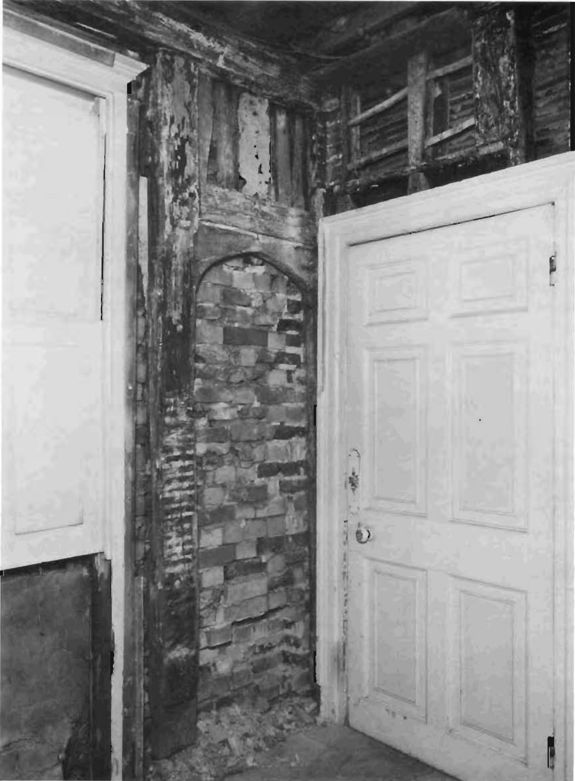
Figure 40 59 High Street, Buntingford, Hertfordshire; photograph of the corner of a room. The photograph readily conveys the nature, materials and form of a rediscovered early doorway formed in the timber frame and subsequently blocked
