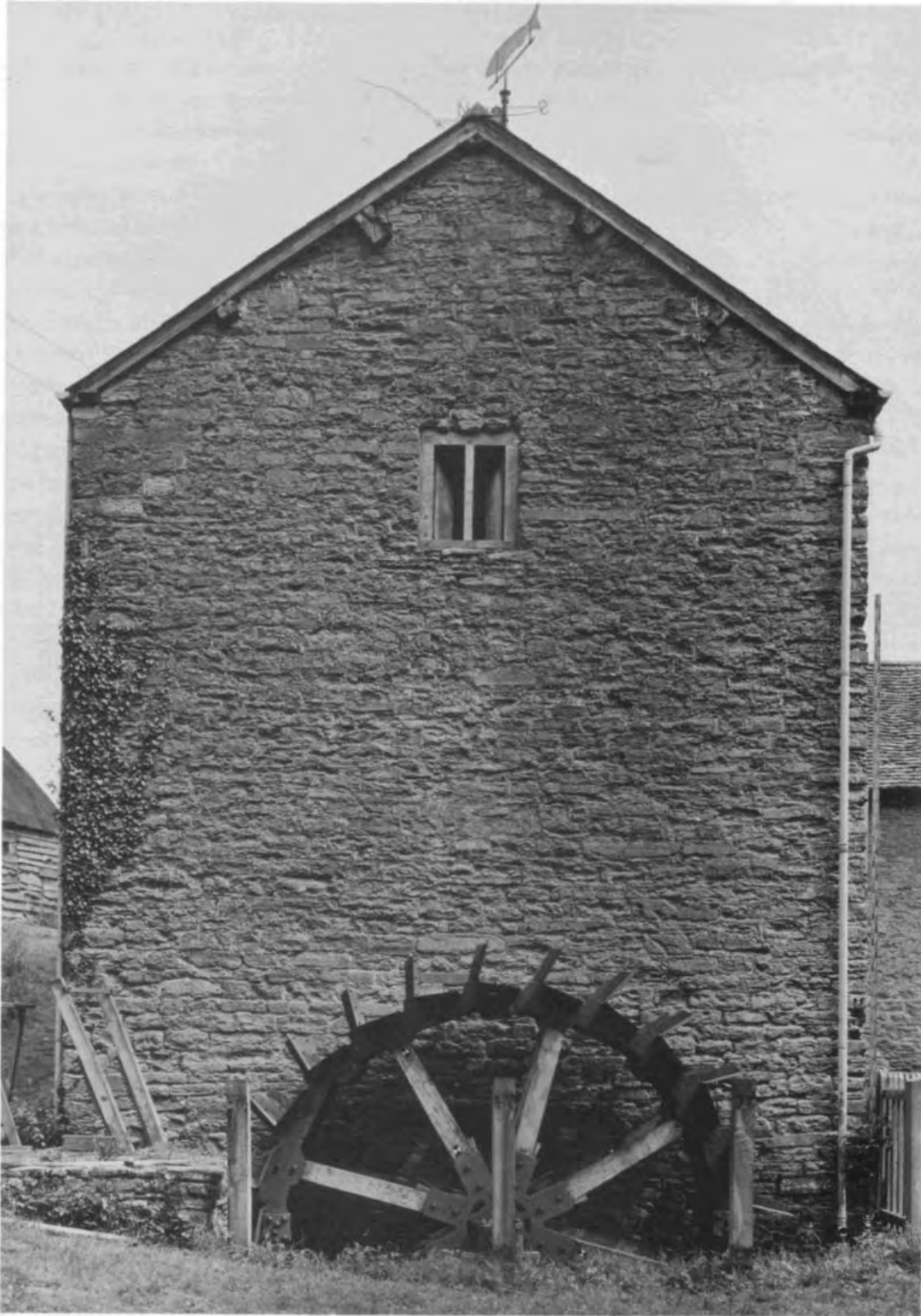
Figure 41 Mortimer's Cross Water Mill, Herefordshire; an elevation recorded by rectified photography. This technique is especially suited to simple rectilinear buildings with few changes of elevational plane. Figure 42 shows that, where a reasonable camera location cannot be found, part of the elevation has to be indicated in another manner
