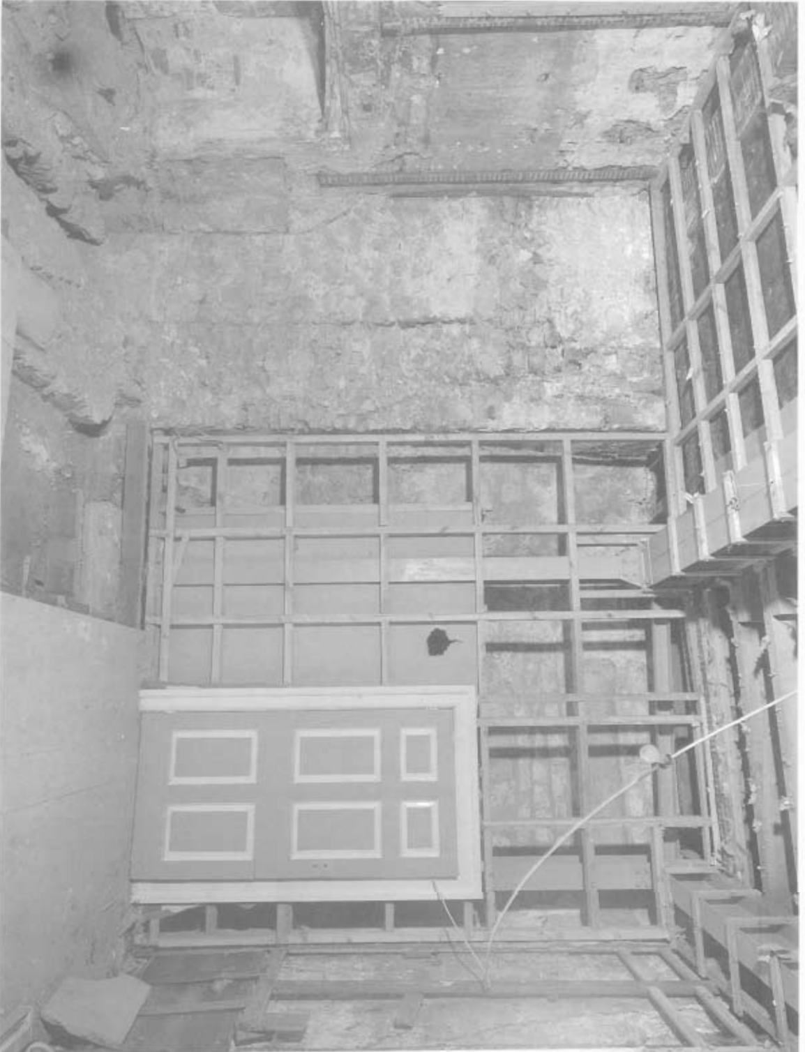
Figure 19 The Archbishop's Palace, Maidstone, Kent; a further example of evidence of earlier structures revealed by removal of wall coverings and excavation of the floor – in this case a sixteenth century fireplace as well as the footings and abutment of a medieval wall
