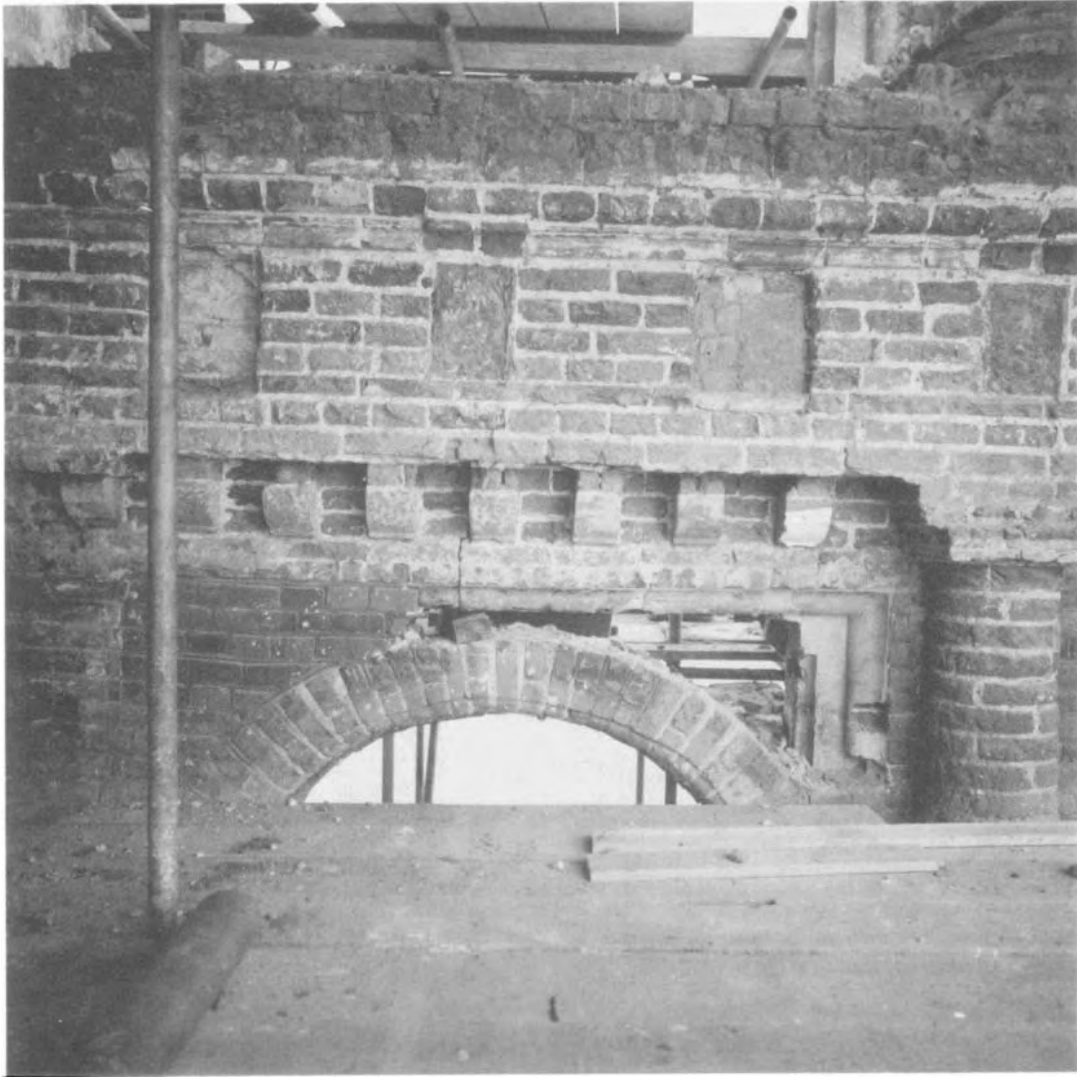
Figure /6 Hill Hall, Epping, Essex; progress photograph showing details revealed by the removal of later material. See also Figures 15 and 17
