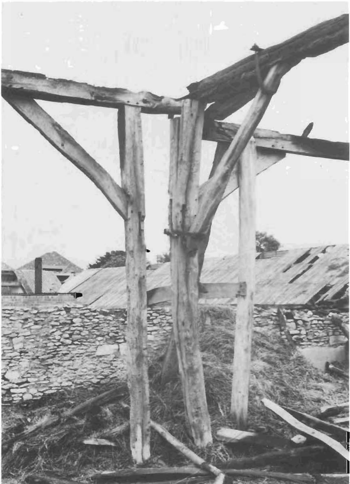
Figure 39 Barn at Walton, Peterborough, Cambridgeshire; photograph of surviving members of the structural frame. To record such a deformed structure by drawing would be practically impossible; the camera records the essential features of the structure and its jointing and assembly
